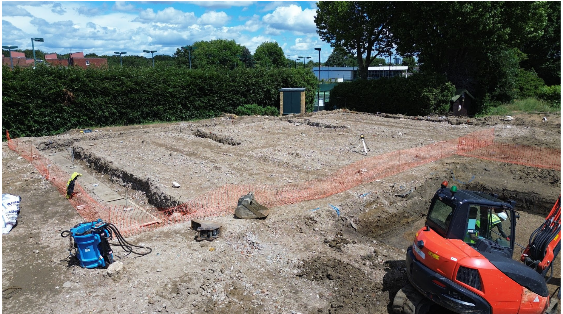
Site of the building from the south east corner.
