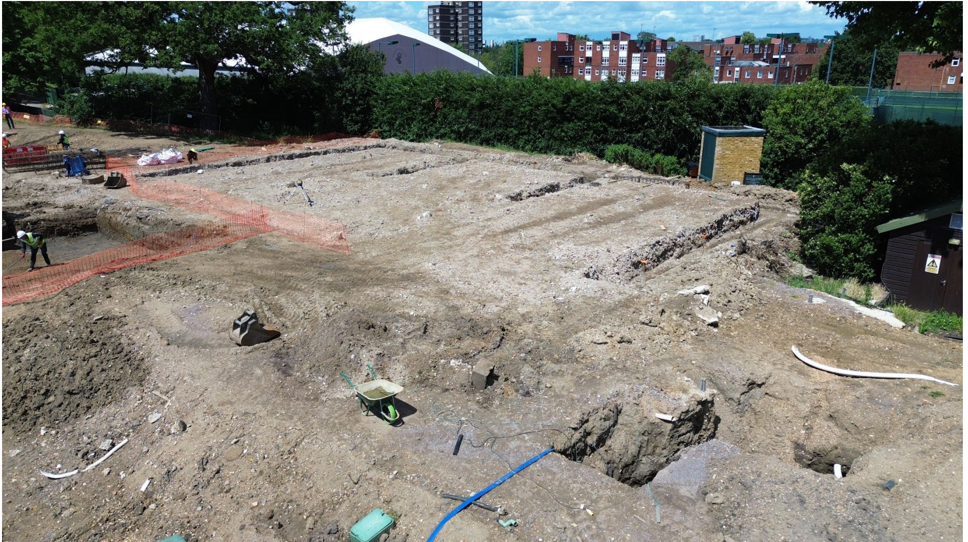
Site of the new building from the south west corner
