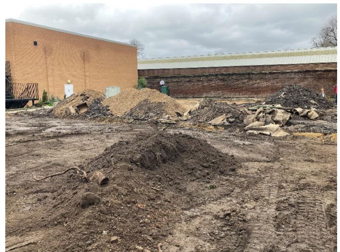
Ground breaking has begun for the new Padel courts
