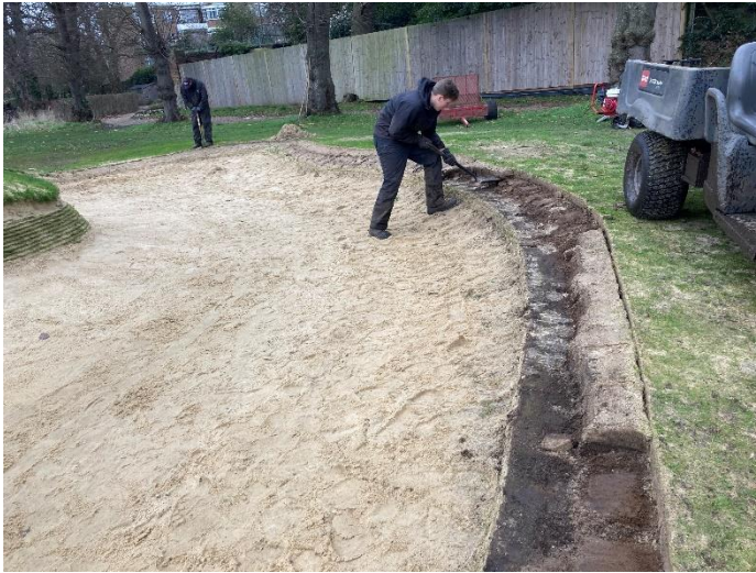
Renewing the edge of our practice green bunker and installing a new revetted side
